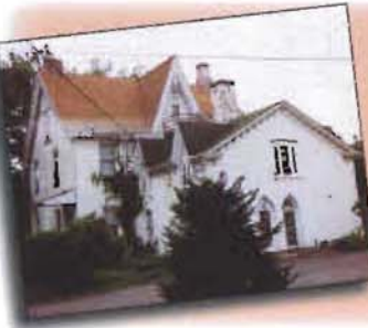
#8 302 Third St., Atty. David Cash Homestead, Gothic Revival, 1846. David Cash served as Bradford County district attorney and prothonotary. Architectural features: Attic level Gothic gables with ornate verge boards; 2nd story window in a lancet shaped arch above triple-arched entrance, trefoil columns.
